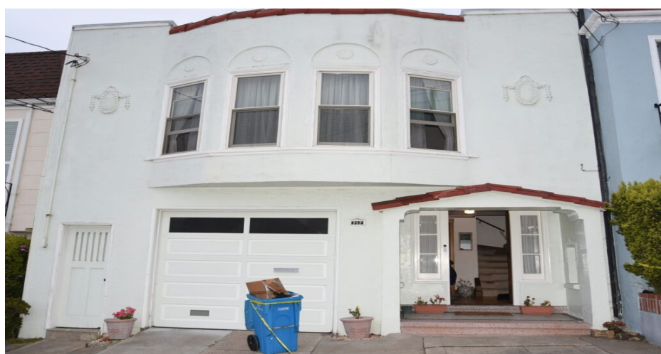
Figure 1- Daytime photo of home on 31 st Avenue, San Francisco, California
